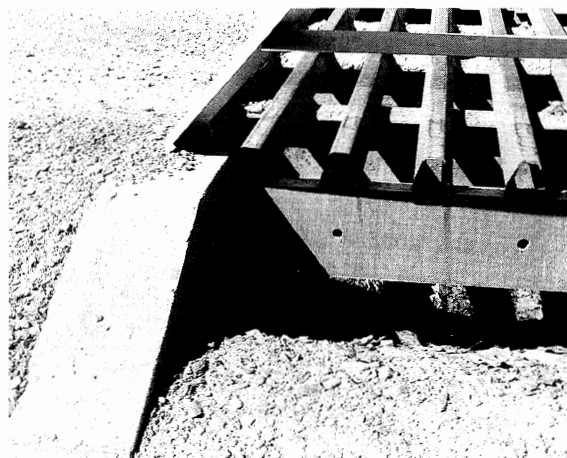
Concrete foundation cattleguard (detail).
