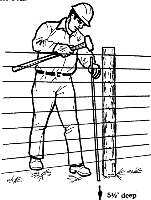
Installing a ground rod.
