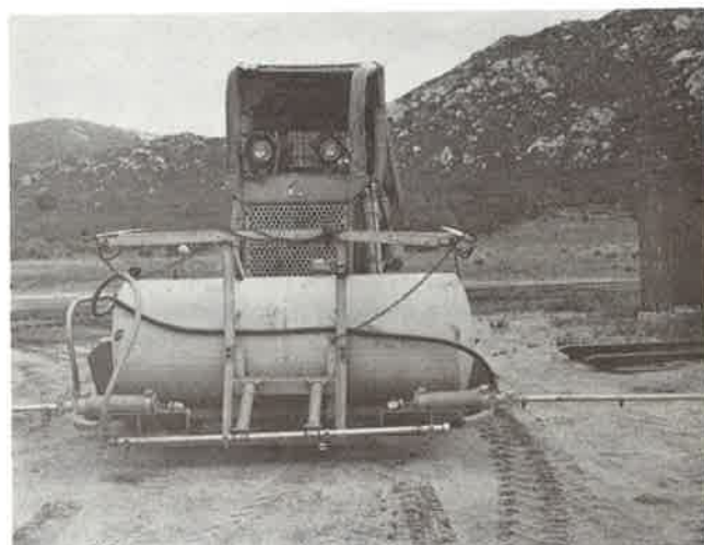
Single-point mounted boom sprayer on a crawler tractor.
