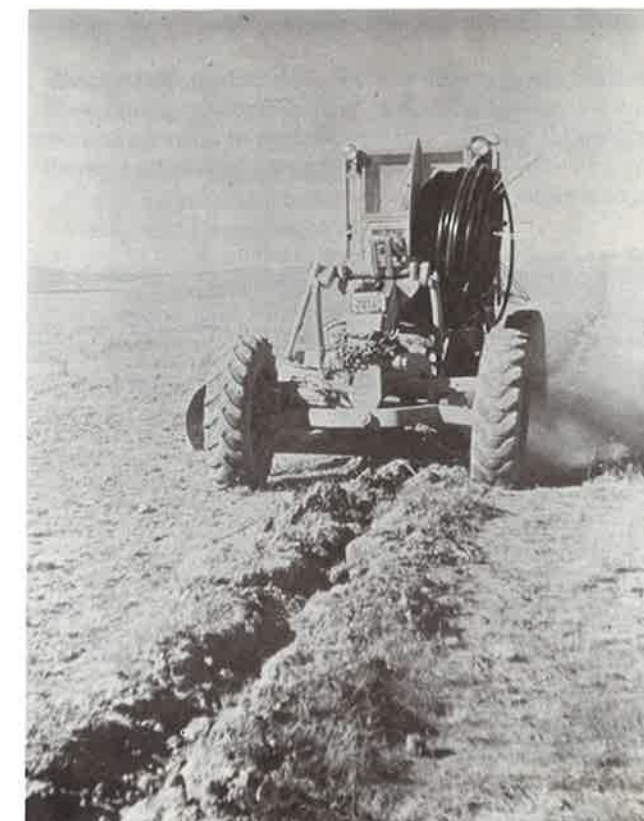
Plastic pipe laying equipment attached to a motor grader.
