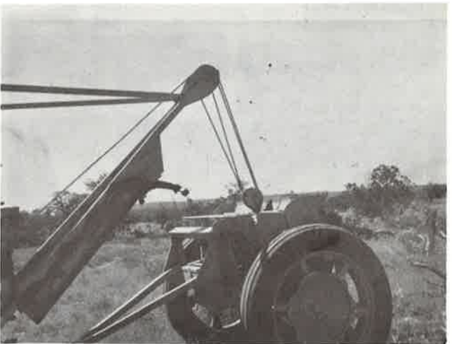
Half-sized rangeland drill mounted on a crawler tractor.
