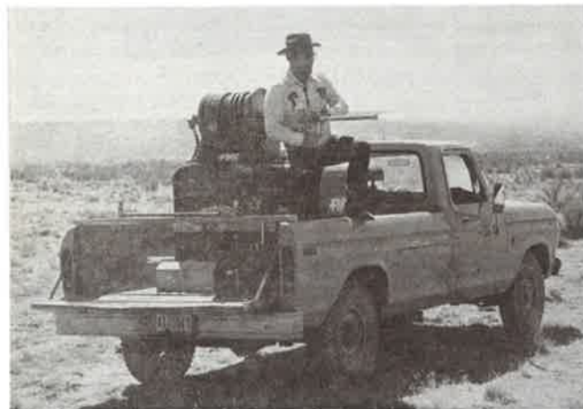
Skid-mounted sprayer with a hose for spot treatments.
