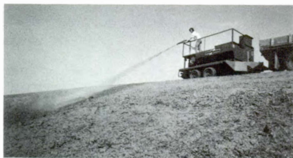
Trailer-mounted hydraulic seeder-mulcher treating a slope.
