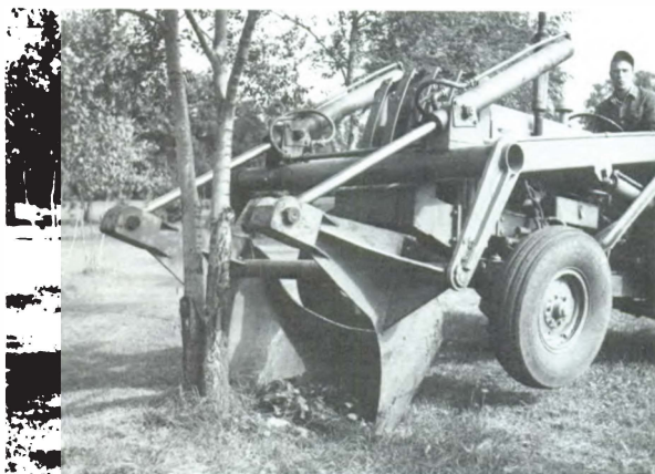
Detachable grubber mounted on a standard dozer blade.
