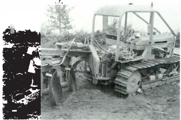
Double-disk contour trencher.
