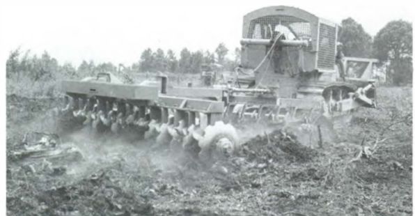
Disking action of the offset disk gangs.
