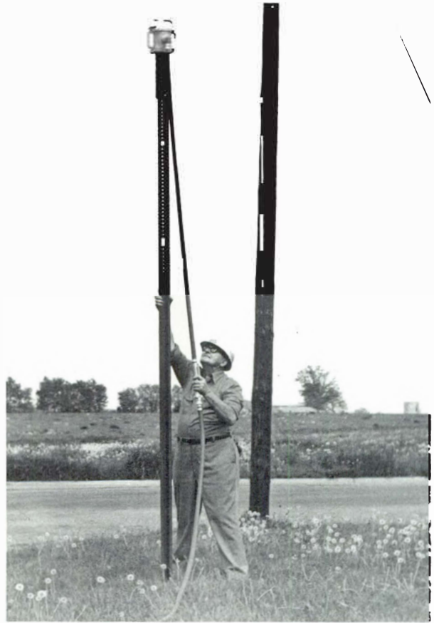
Air-powered post driver.
