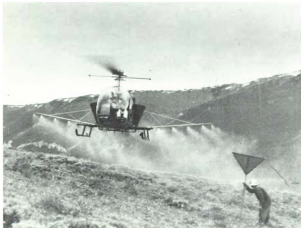
Helicopter boom sprayer with side tanks.
