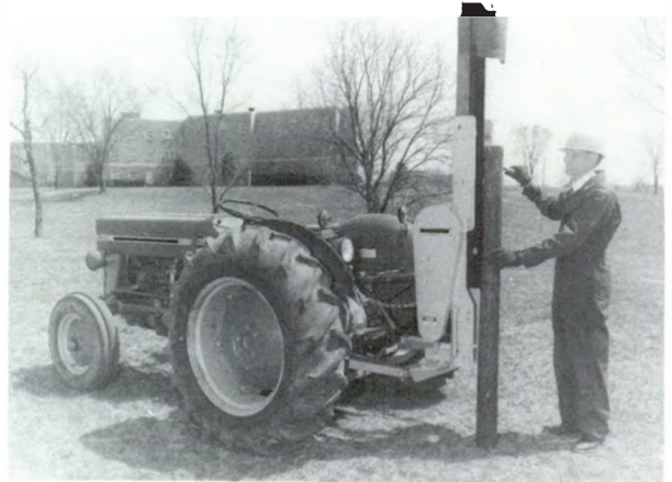
Power-take-off post driver mounted on a three-point hitch.
