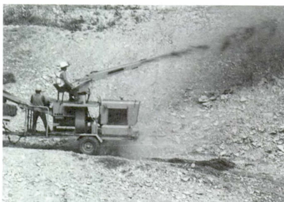
Power mulcher treating a steep slope.
