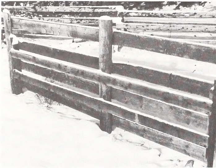
Guardrail allows livestock to be worked on both sides of fence
