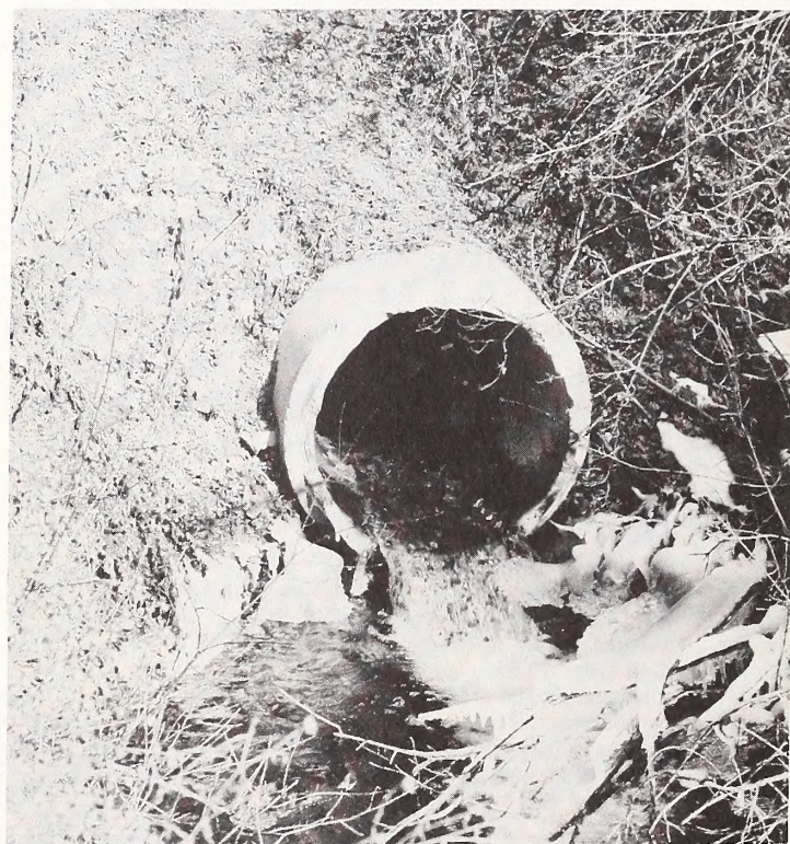
Concrete culvert
