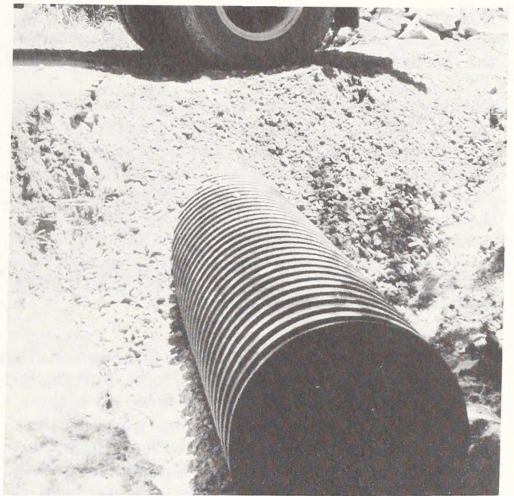
Polyethylene culvert
