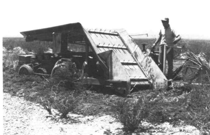
Brush pickup conveyor on New Mexico State University demonstration arid land seeder.
