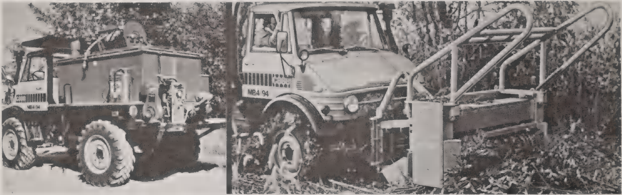
Case Unimog designed for forest firefighting reforestation, and land clearing is equipped with 500-gallon Pacific pumper and Royer shredder.
