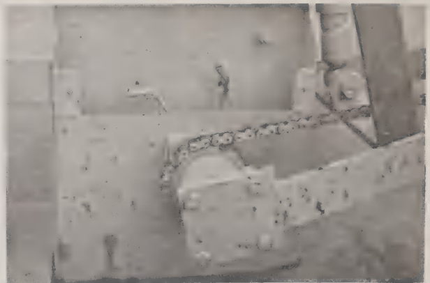
Backside view of thimble seeder showing spokes with thimbles attached.
