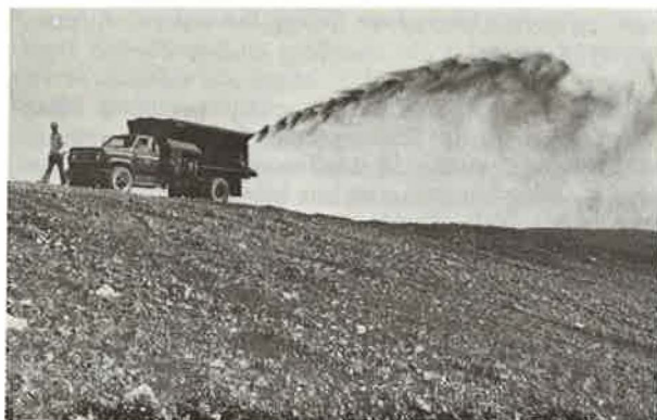
Bark mulch is being applied on a surface mine site with an Estes Spreader.
