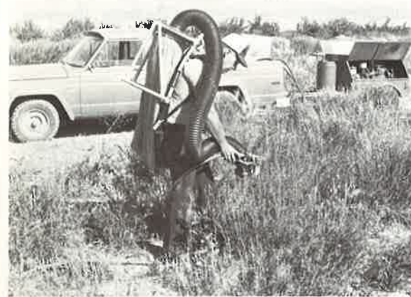
Collecting forb seeds at Ephraim, Utah, with air amplifier seed collector.
