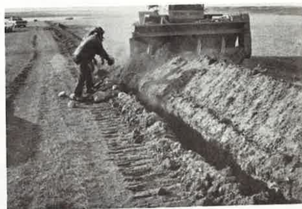
Figure 4.—Rocks dug out by the trencher are safely returned to the trench because the fine material has already covered the pipe.
