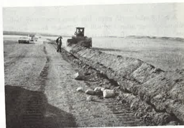
Figure 3.—Earth auger backfilling pipeline trench at 1 mph.
