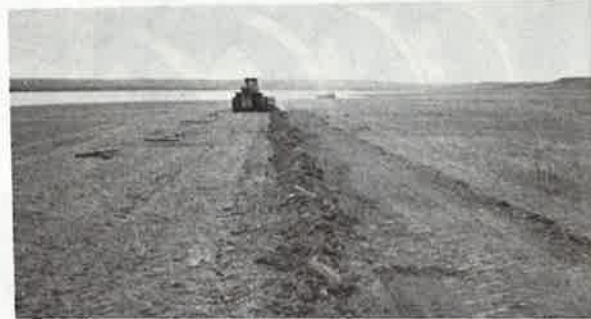
Figure 4.—Rocks dug out by the trencher are safely returned to the trench because the fine material has already covered the pipe.
