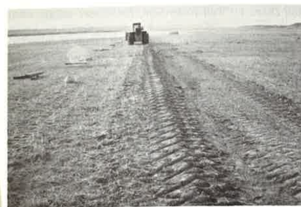
Figure 6.—Operator uses tire to pack down material, eliminating crown and speeding consolidation.
