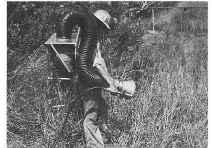
Figure 1.--Backpack-carried 8-inch air amplified seed collector.
