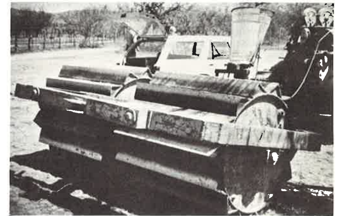
Converted sheepfoot roller imprints a 9-foot width.
