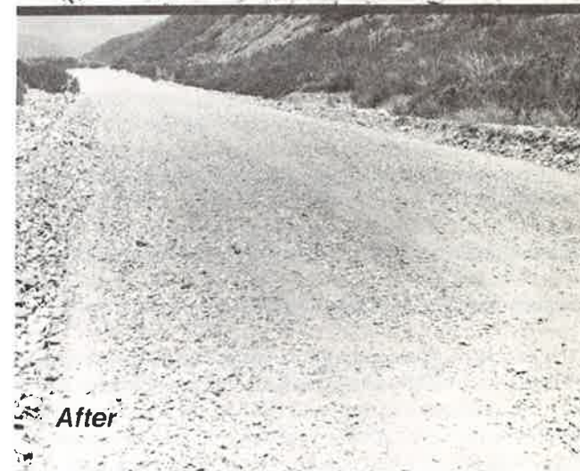
Road before and after treatment by mobile hammermill.
