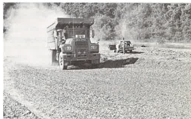
Dust plumes stirred by coal truck as it passes from untreated segment of haul road onto section treated with wood chips.
