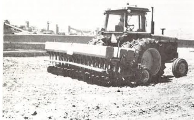
A tye drill seeds land disturbed by strip mining near Farmington, N. Mex. This drill can seed three different types of seed and dispense fertilizer at the same time.
