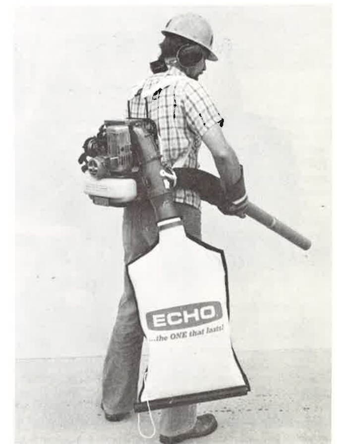
Echo PB-400 power blower with vacuum attachment that can be used as a backpack seed collector.
