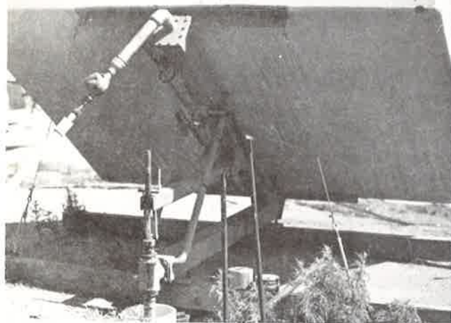
Solar-thermal water pumping system operating near Tucson, Ariz.
