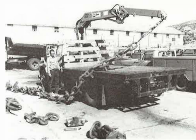
Truck used to transport chain. A crane-equipped truck has proven to be very effective in transporting the chain and maneuvering it to weld on digger teeth and change swivels and clevis connection.
