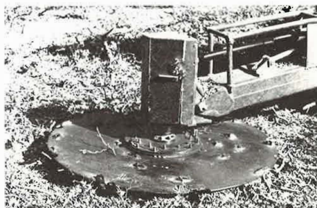
SHAR "Twenty" cutter head: 6-foot disk with cutter teeth.
