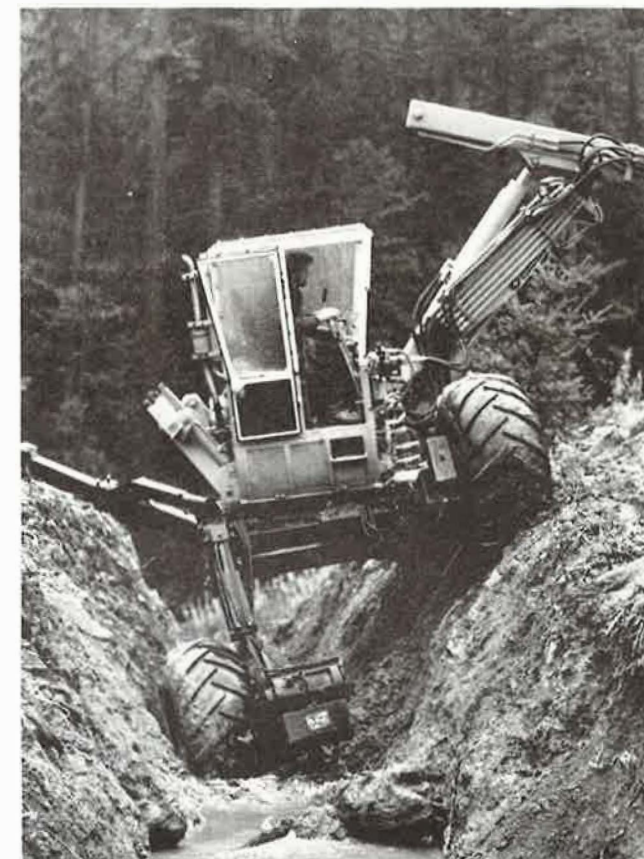
The Center's Menzi Muck 5000 T2 excavating to drain sag ponds on a landslide.
