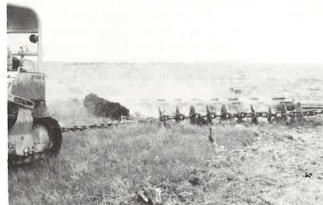
Triangular disk-chain developed to prepare seedbeds on extensive areas of log-littered rangeland.
