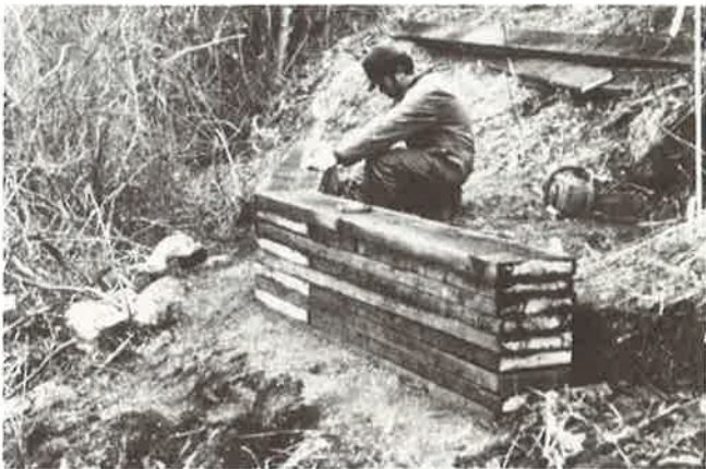
Figure 1.—West abutment during construction.
