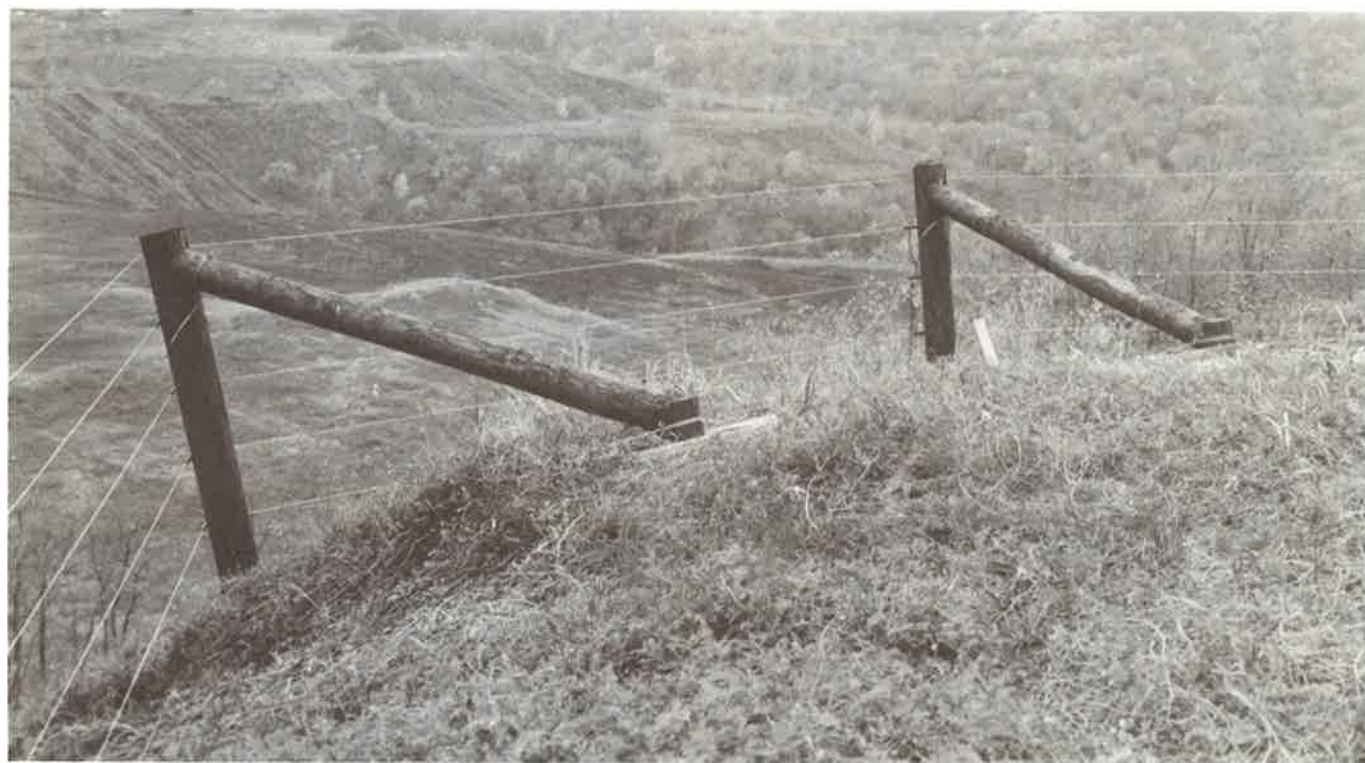
Figure 11.—Diagonal strainer in use at a dog leg.
