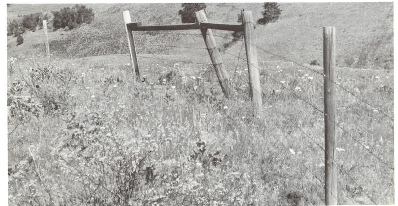
Figure 1.—Fence failure at dog leg.
