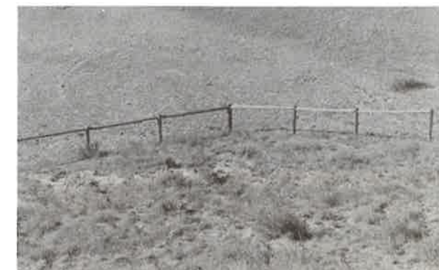
Figure 9.—Using a six panel strainer assembly to increase the effective length of a strainer beyond the critical length at a dog leg.
