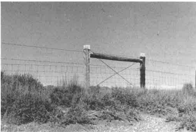
Figure 4.—Conventional horizontal line strainer.
