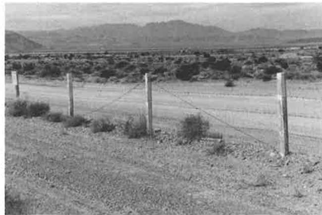
Figure 5.—Tension member line strainer.
