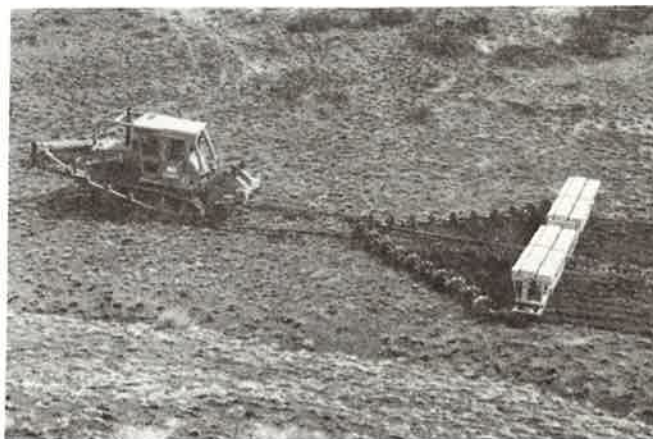
D-7 caterpillar tractor pulling a disk chain. A 30-foot wide swath is seeded by this disk chain.
